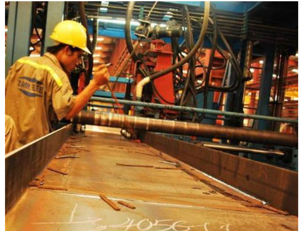
Flawless full penetration weld for flange to web connection
