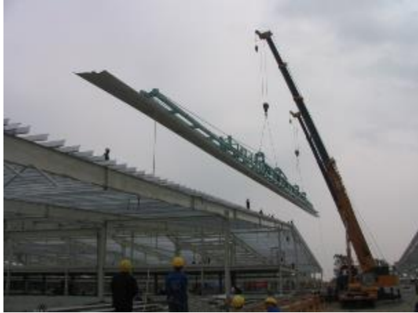
Hoisting of Panels to Roof
