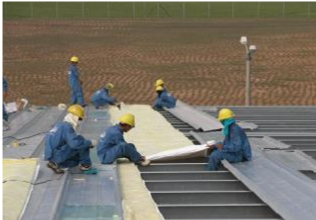
Installation of Insulation and Laying of panels
