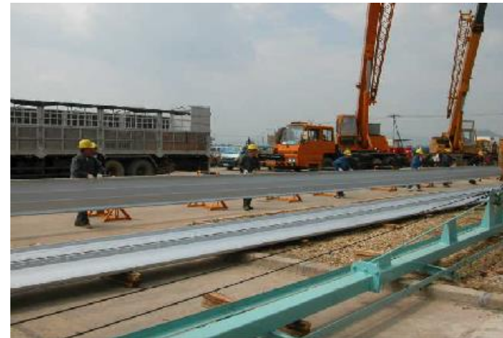
Unloading Panels for Hoisting
