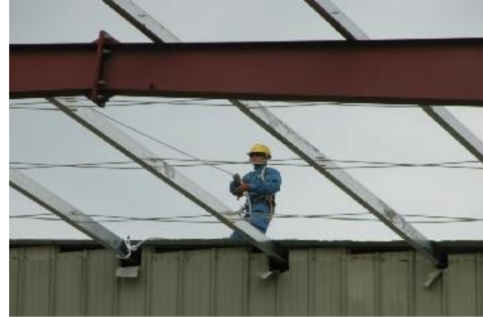
Spreading Panels on Roof
